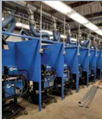
Welding Facility — A metal building on the Pensacola campus was remodeled for use by the College's welding program.
