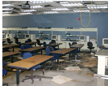
Classroom damaged by Ivan.
